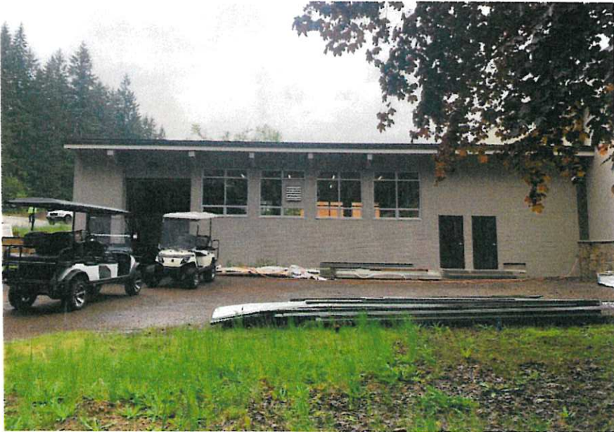
Exterior view of the shop which is an original structure. Construction of the new community center and City Hall was done from 2021-2022 but did not change this original structure, aside from external painting. The proposed project is to install a catering kitchen in a portion of this building which is the original shop.
