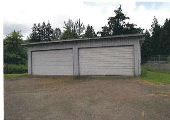
Figure 5.4. Accessory garage building
