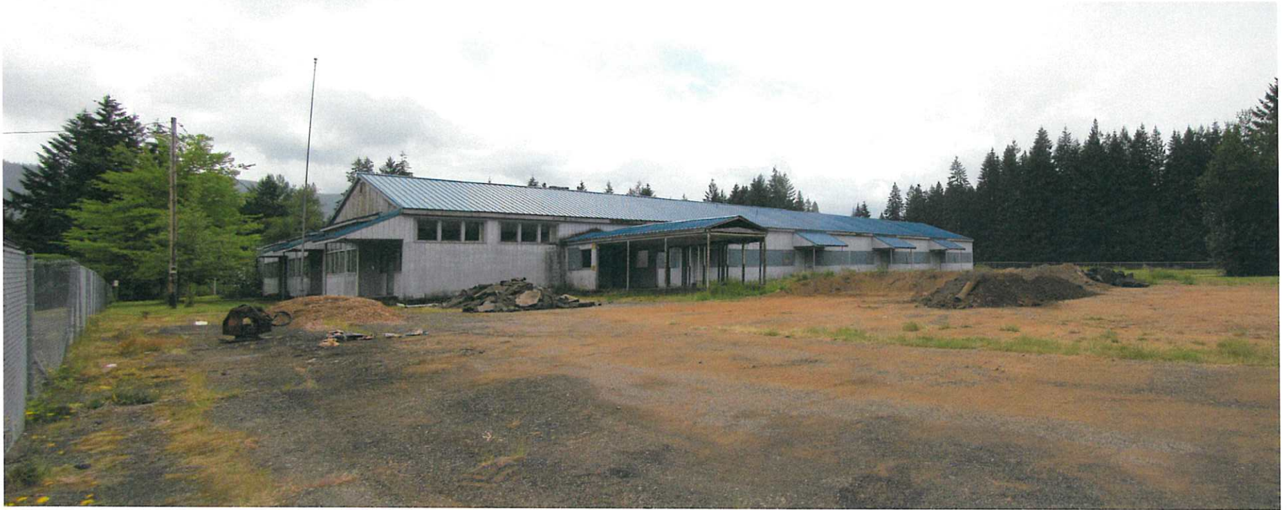
Figure 1. View of existing site
